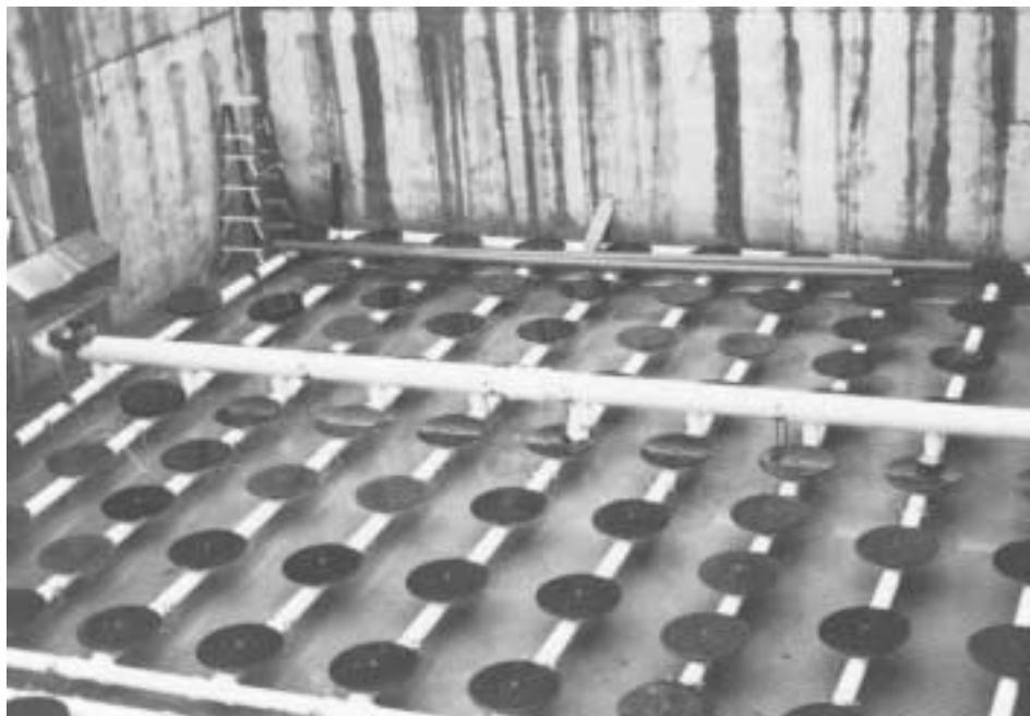
Figure 8-38(f) Alternative device for diffusion: Disk diffuser. (Photo courtesy of U.S. Filter/Envirex.)
