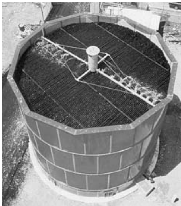
Figure 8-45(a) Aerobic fixed film systems; trickling filter. (Photo courtesy of NSW Corporation.)
