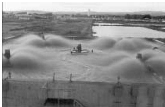
Figure 8-38(o) Alternative device for aeration: Sequencing batch reactor (SBR). (Photo courtesy of Paques ADI Systems, Inc.)
